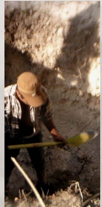
The septic 'tank' being dug with a shovel.
