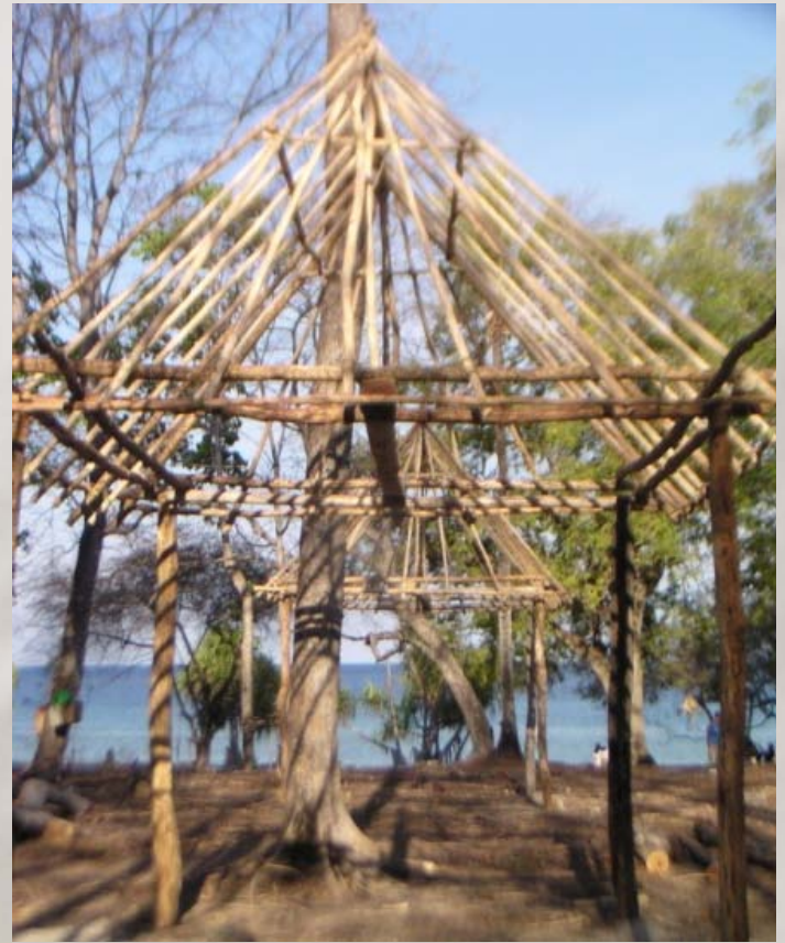
The frame of two of the lodges made of bush timber and fastened with rattan strings
