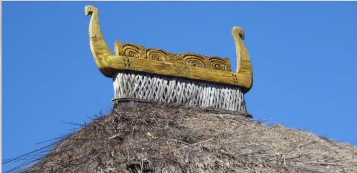
A typical roof top of a uma lulik in Maubara
