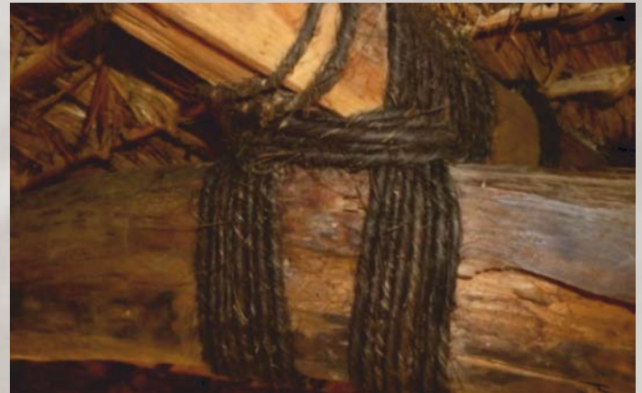
Ropes made from the aren fibre used as fasteners for beams in buildings
